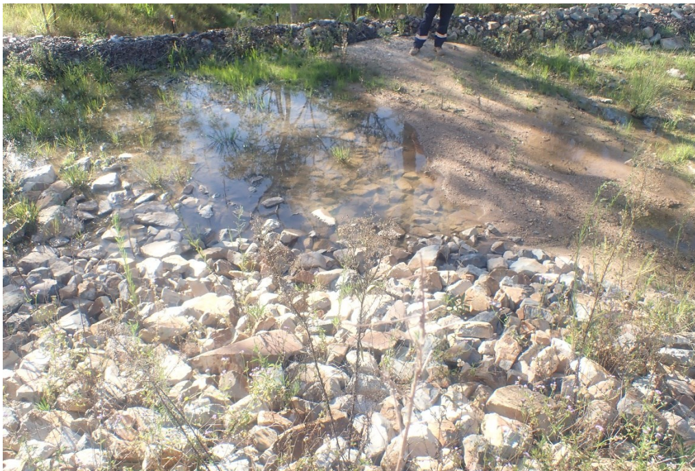
Plate 21: Sediments building up within the large sediment trap at Impact Site 2
