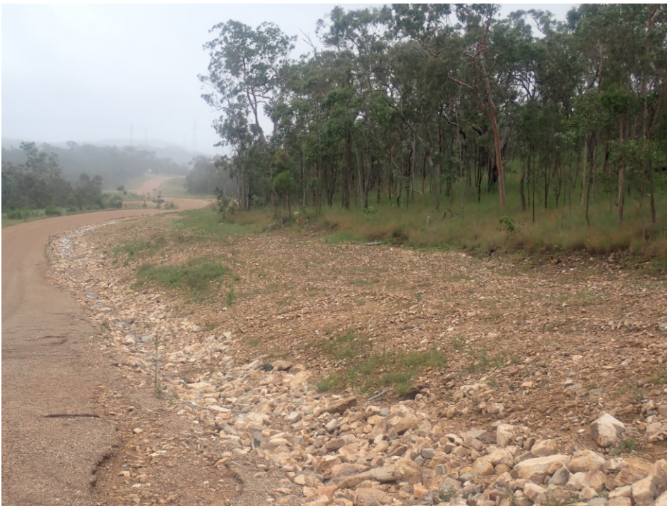
Plate 4: Minor sheet and gully erosion on roadside verge between Four-Ways intersection and WTG09, on granitic soils.
