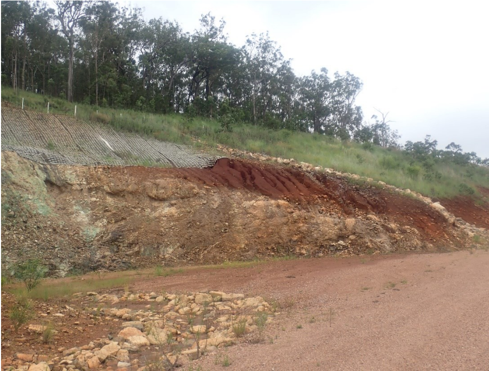
Plate 4: Minor sheet and gully erosion on roadside verge between Four-Ways intersection and WTG09, on granitic soils.
