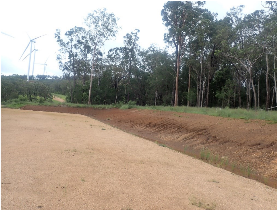
Plate 2: Moderate gully erosion on basalt soils at WTG17.
