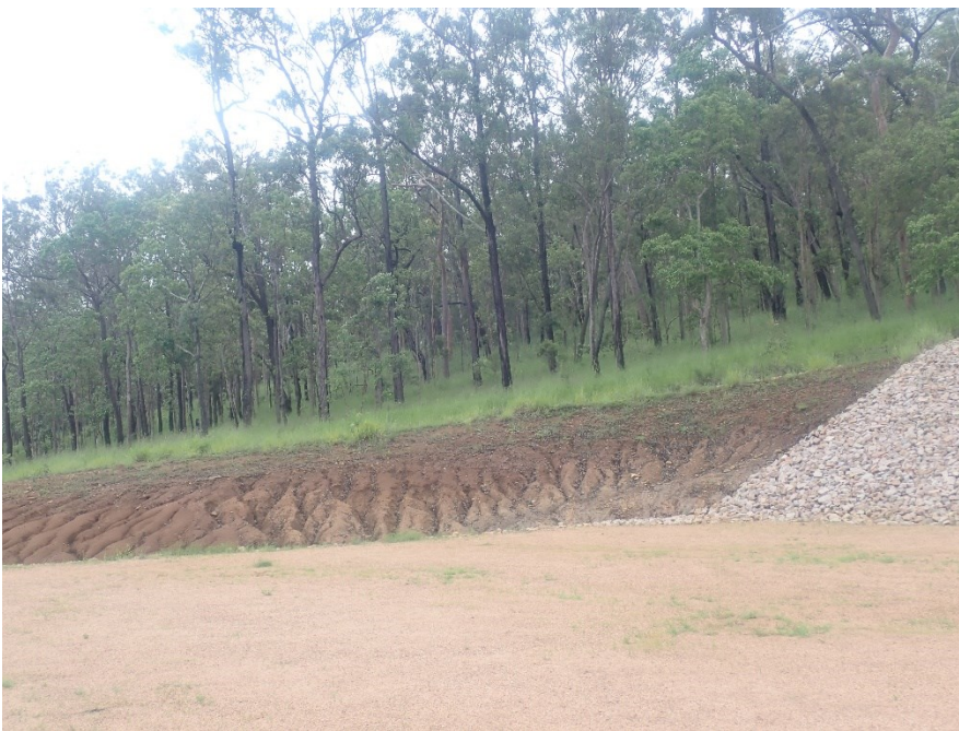
Plate 2: Moderate gully erosion on basalt soils at WTG17.
