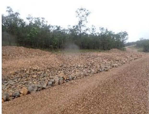
Plate 6: Rock-lined drainage on eastern side of road
