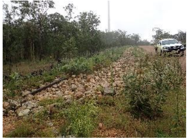
Plate 32: Roadside rock-lined drainage
