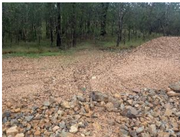
Plate 8: Sheet and gully erosion beginning to form
