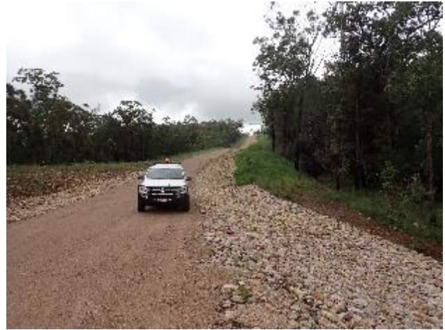
Plate 21: Rock-lined drainage install
