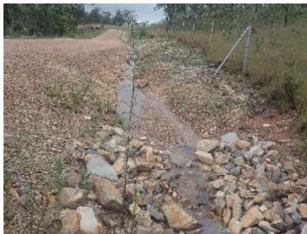
Plate 14: Small rock checks installed on the southern roadside with some sedimentation present
