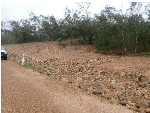
Plate 7: Additional image of rock lined-drainage upgraded from previous years
