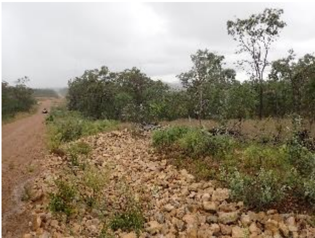
Plate 33: Additional image of Roadside rock-lined drainage
