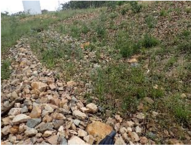
Plate 20: Rock-lined drainage with some sediment accumulation and weeds present
