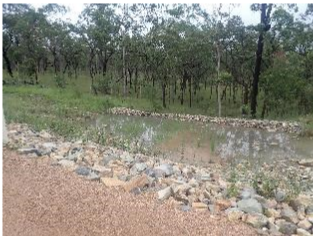
Plate 13: Sediment trap with some sedimentation present and water pooling after recent rain
