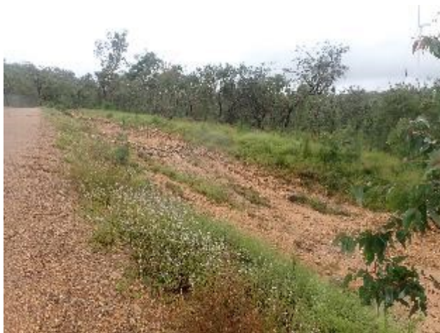
Plate 5: Rock checks installed on western side of road
