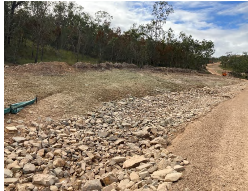
Rock-filled roadside drainage and large rock filled sediment traps
